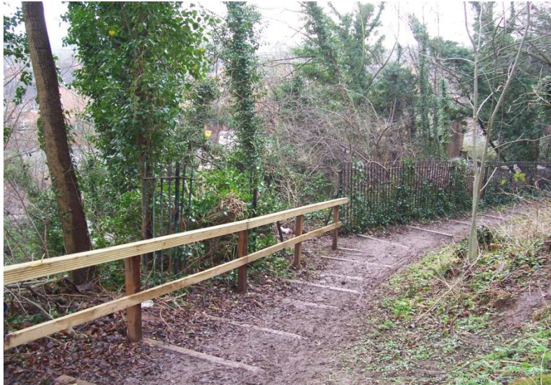
Figure 6: (after) handrail and sleeper steps have been installed along the steepest section. This has improved the overall accessibility of the path and reduced runoff and erosion
