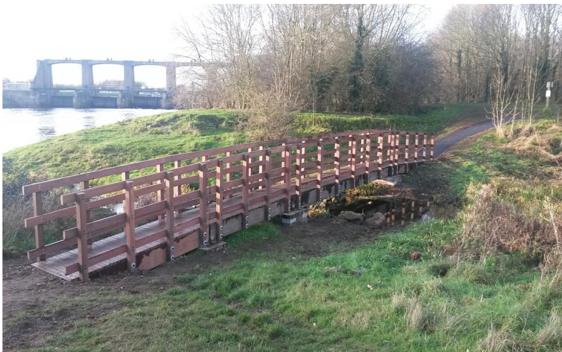
Figure 7: footbridge at Colwick Country Park
